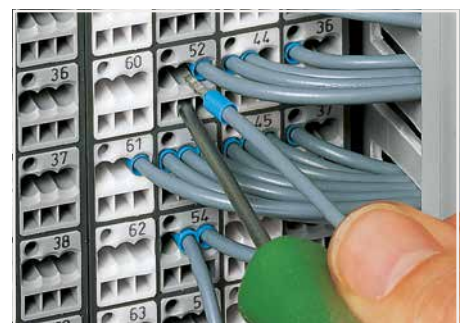
Terminating ferruled conductors via operating tool.
