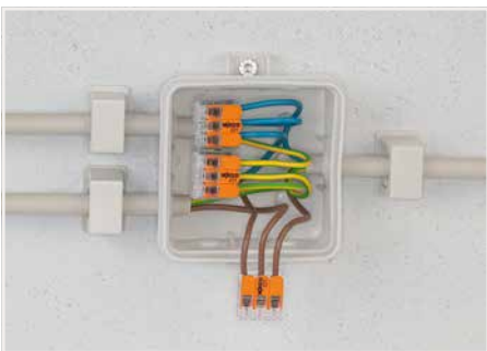
Wiring fine-stranded conductors in a junction box.
