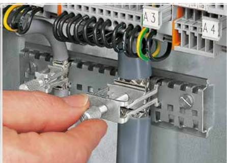
Tightening/removing a shield clamping saddle.
