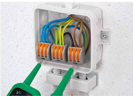
Testing the wired connectors.
