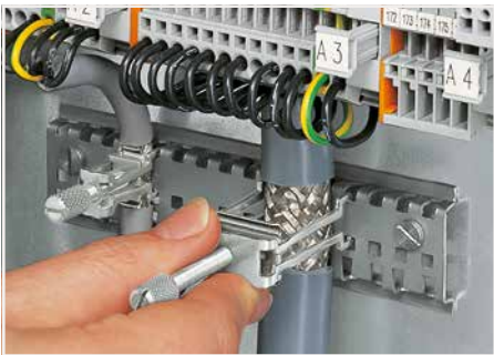
Securing an additional shield clamping saddle.
