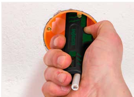
Stripping a cable sheath.
