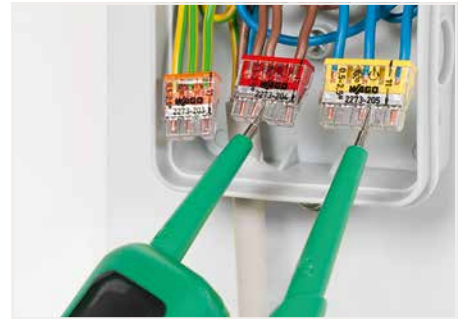
Testing via test port opposite to conductor entry.
