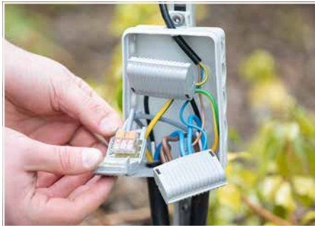
Connecting a bollard light
