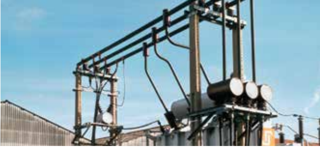
GASLINK® SF 6 insulated busbar system
